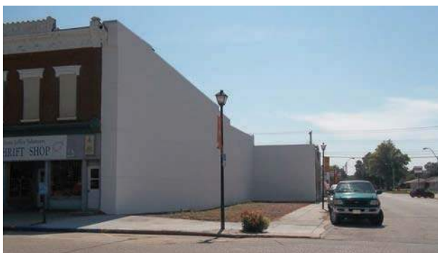
Looking Southeast, Downtown Square - Existing
